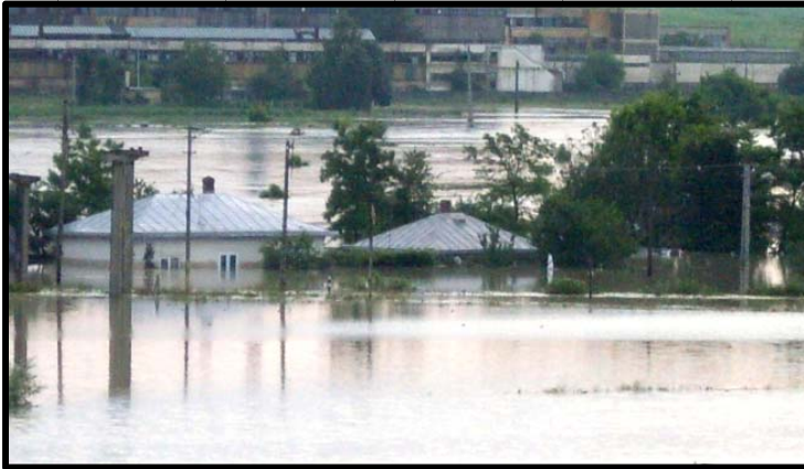
Water, water...everywhere! Houses are almost entirely engulfed.
